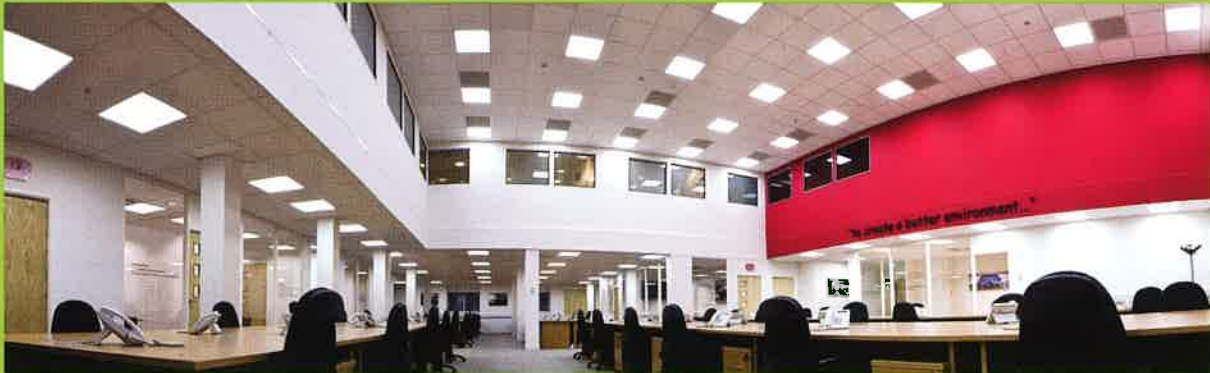
Free standing mezzanine floor with ground and first floor office accommodation.
